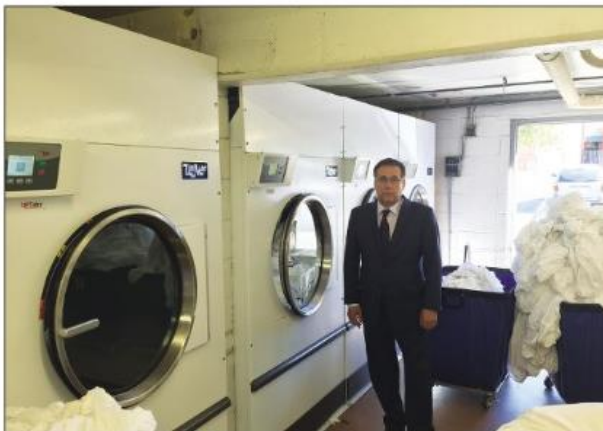
Hotel owner Bruce Rahmani says moisture-sensing technology in his new dryers keeps him from worrying about scorching sheets. (Photos: Alliance Laundry Systems)
